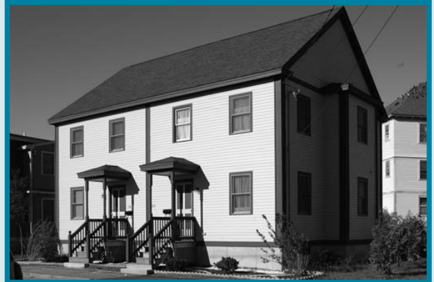
Newly renovated multi - family homes
